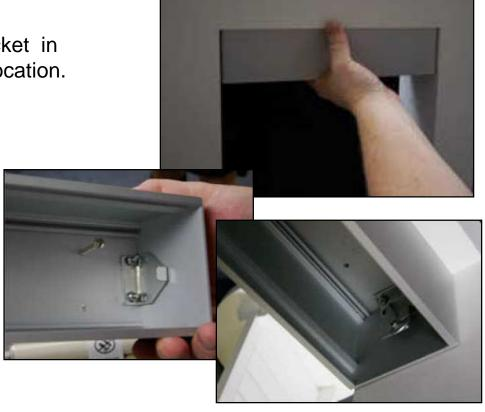
2.Install the side channel backs. The side channel back should abut the pocket, flush with the end plate. Screw the backside channel directly into the window jam.
